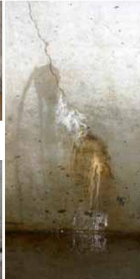
Construction defects (rock pockets, honeycombs & untreated tie holes)
